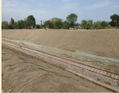
Installation of JGT
