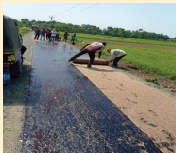
Laying of JGT on treated surface
