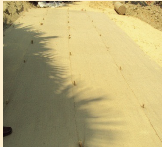
Laying of JGT
