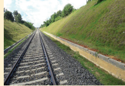
Slope Stabilized with Vegetation
