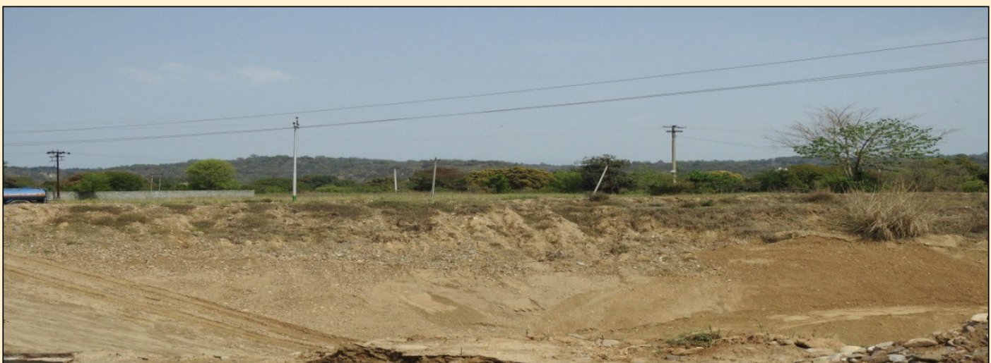
Destabilized slope
