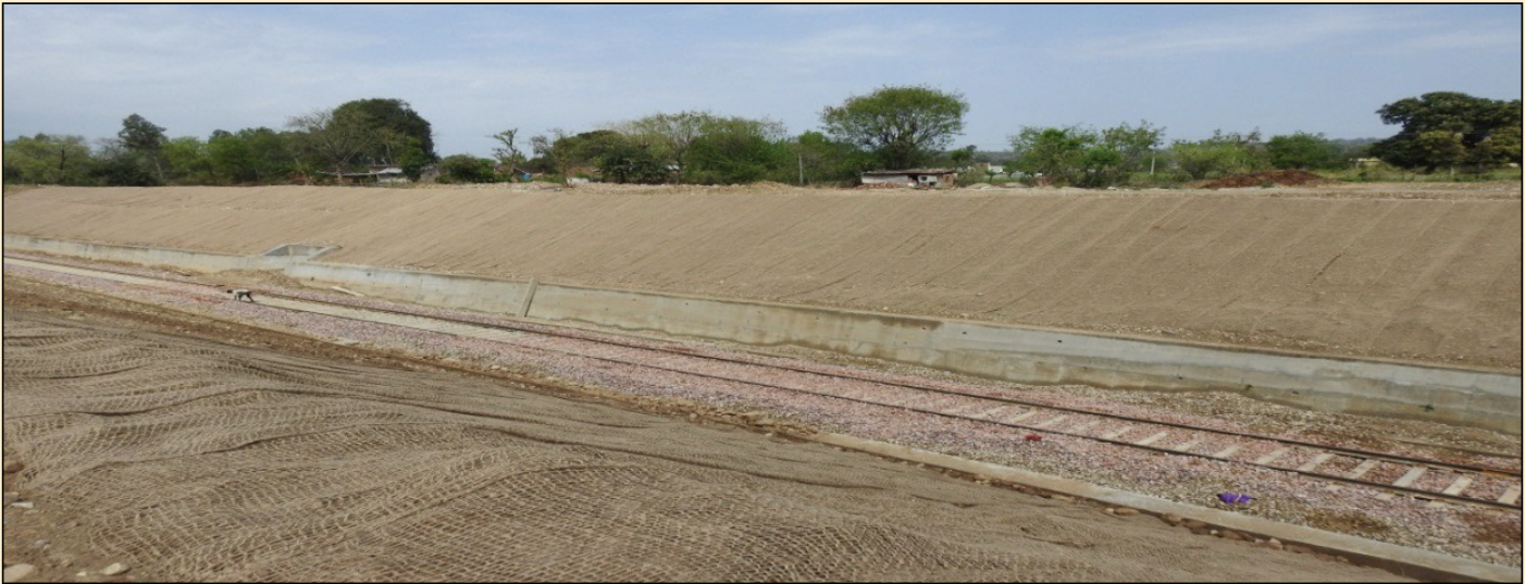
JGT laid over the prepared slope
