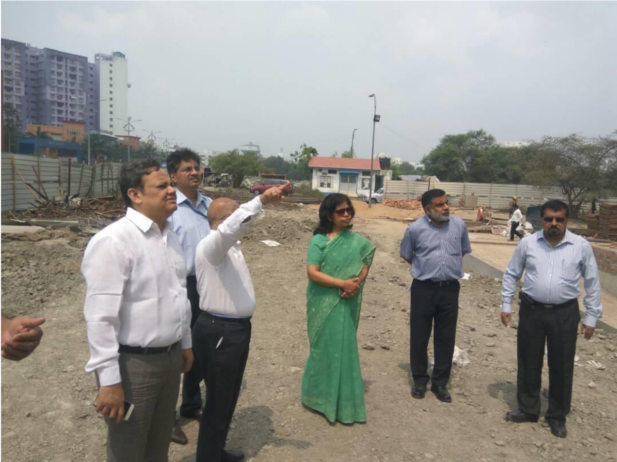
Chairperson NJB and Union Textiles Secretary madam Smt. Rashmi Verma, Visit to the construction site of Patsan Bhavan at Rajarhat Kolkata on 19th April 2017
