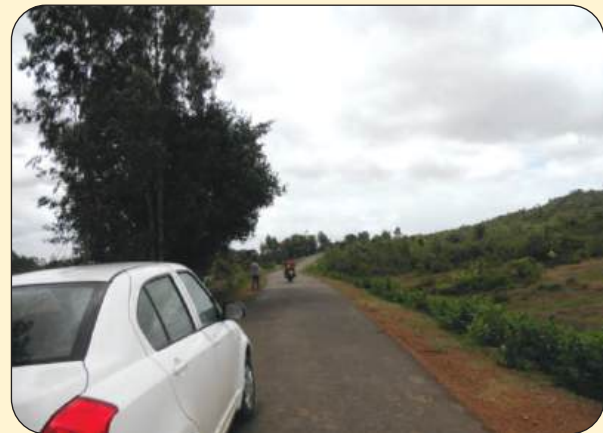
Finished Condition of road after 1 1/2 year (2015)
