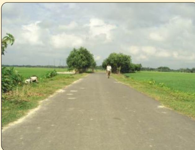
Finished Condition of road after 3 years (2015)
