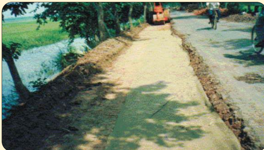
JGT laid over sub-grade
