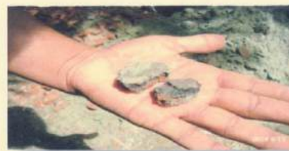
Fig: Condition of JGT during 2nd monitoring
