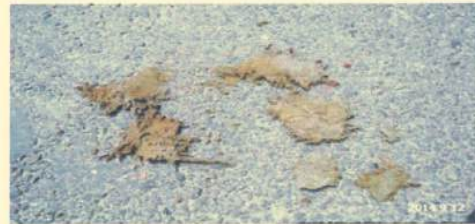
Fig: Condition of JGT during 2nd monitoring
