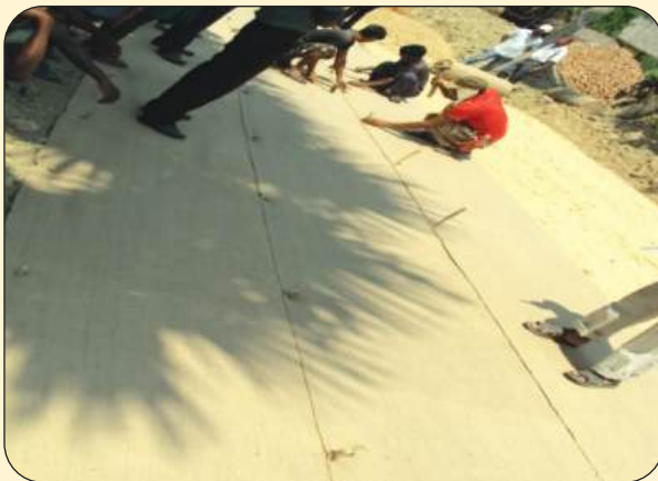
Pegging of overlapped sections of JGT
