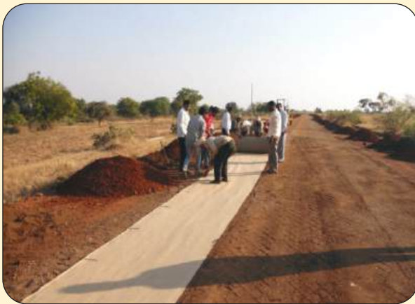
Laying of JGT
