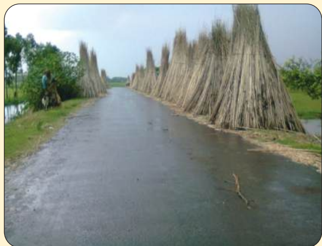
Finished Condition of road after 2 years (2015)
