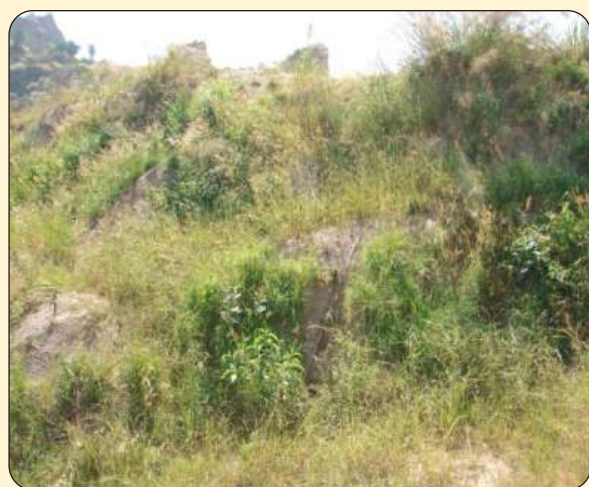
Plantation through JGT laid on slop
