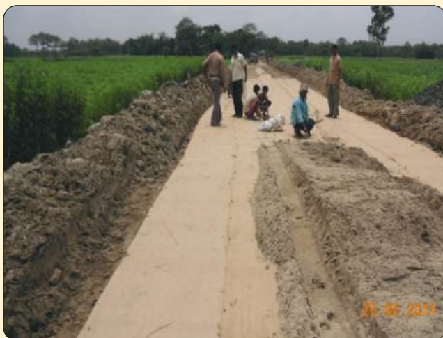
Layer of sand spread over JGT
