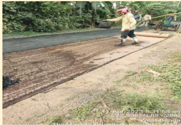
Spreading Prime & Tack Coat on JGT
