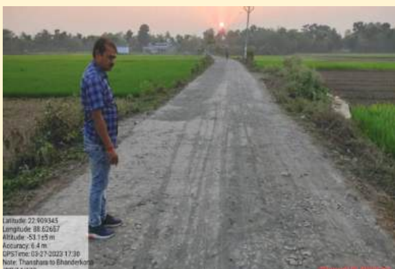
Repaired surface of damaged road
