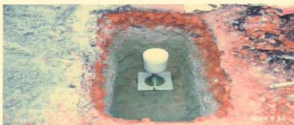
Fig: Performing Field density test during 2nd monitoring
