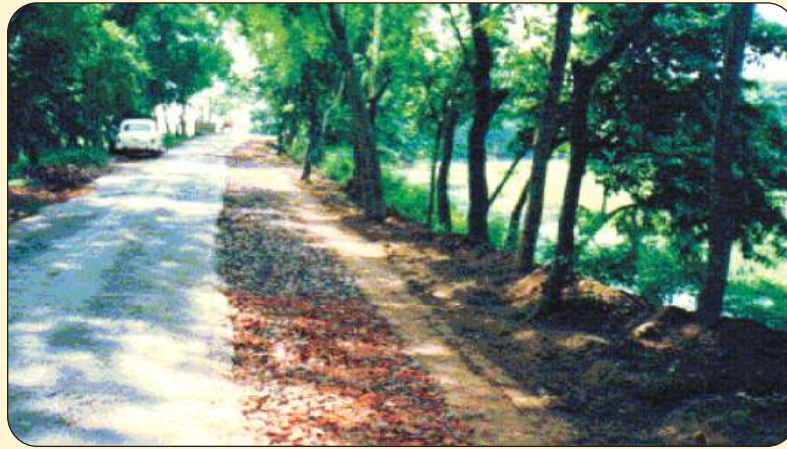
Brick metal laid over JGT
