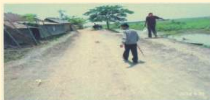
Fig : Finished subgrade
