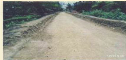
Fig: Condition of road during 1st monitoring
