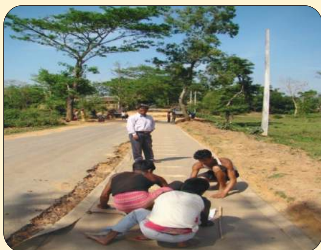
Laying of JGT in widened portion
