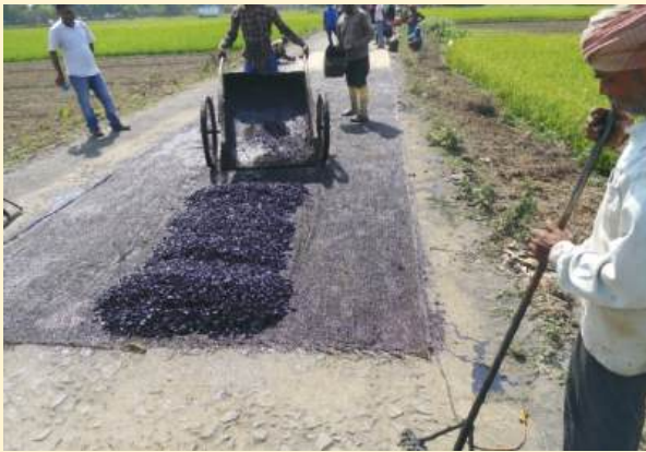
Premix Carpeting on one side of carriage way
