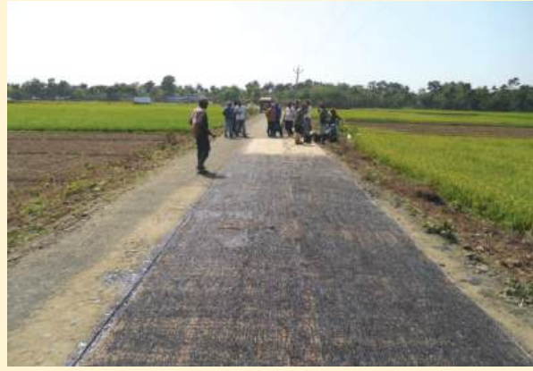
Spreading Prime & Tack Coat on JGT
