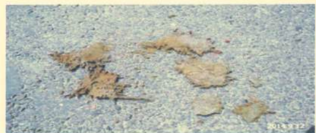
Fig: Condition of JGT during 2nd monitoring
