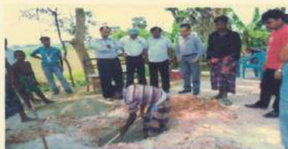
Fig: Field Density test during 1st monitoring
