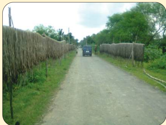
Finished Condition of road after 1 year (2015)
