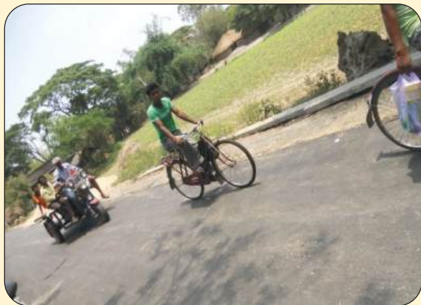
Finished Condition of road after 1 year (2015)
