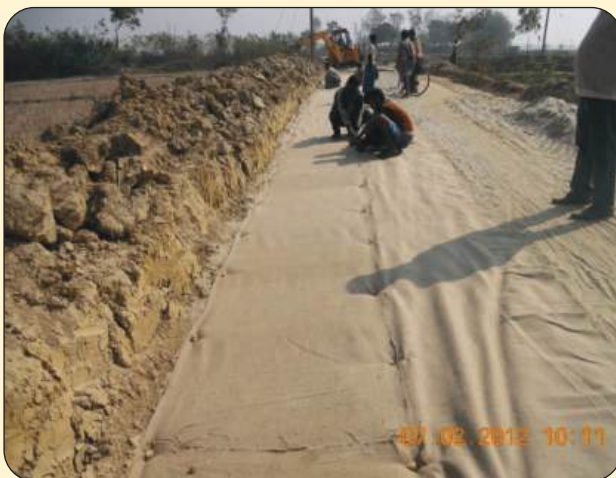
Pegging of overlapped portions of JGT
