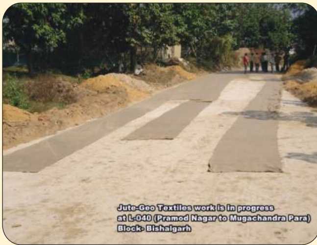
Laying of JGT
