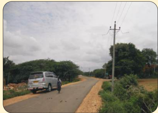
Finished Condition of road after 1 1/2 year (2015)
