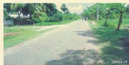
Fig: Condition of road during 2nd monitoring
