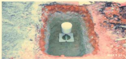
Fig: Performing Field density test during 2nd monitoring
