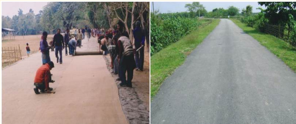
VIEW DURING LAYING OF JGT & FINISHED CONDITION ROAD AFTER 23 MONTHS
