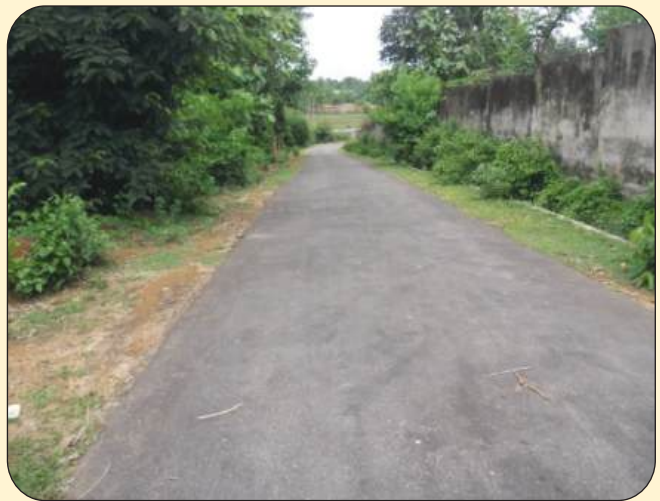
Finished Condition of road after 2 years (2015)
