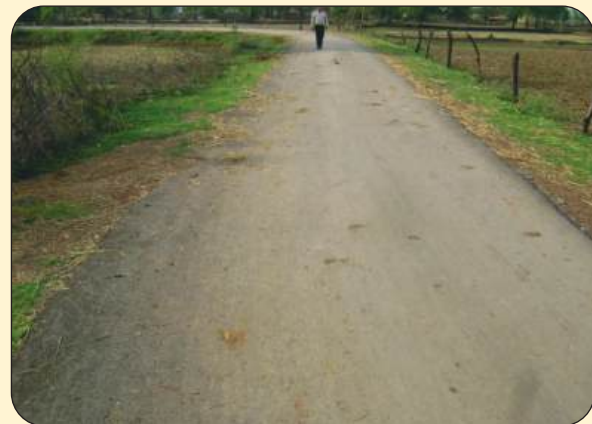
JGT laid section after 26 Months (2009)
