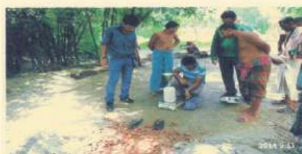
Fig: Field density test during 2nd monitoring
