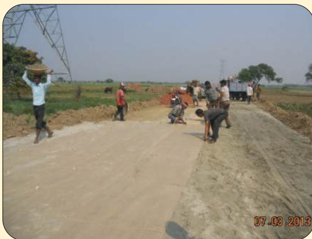
JGT laid over sand
