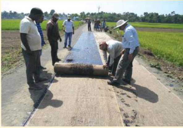
Laying of JGT
