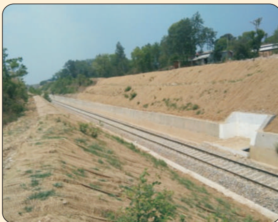
Sprouting of grass seeds through pores of JGT
