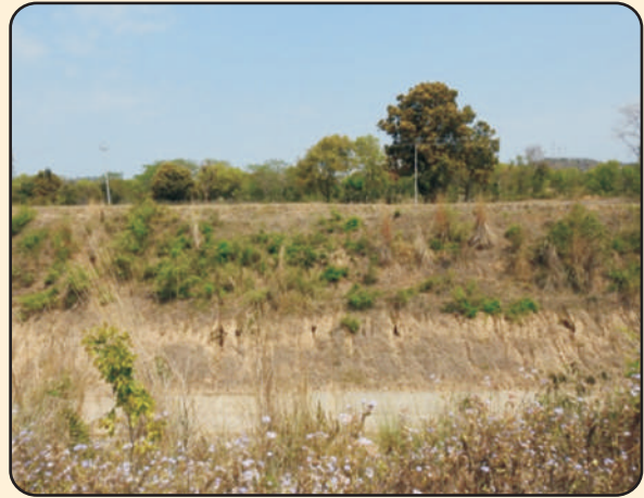
Eroded Slope of Cuttings
