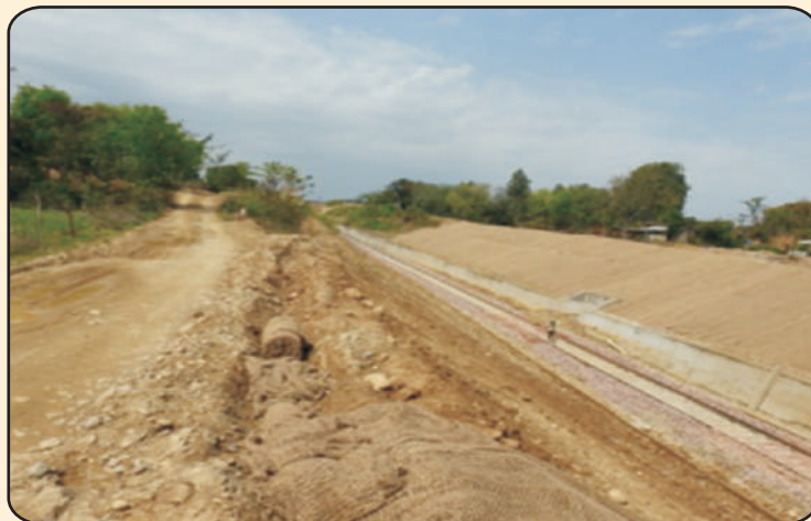
Dressing & Installation of JGT
