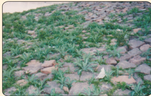
View of condition river bank after three years of JGT application
