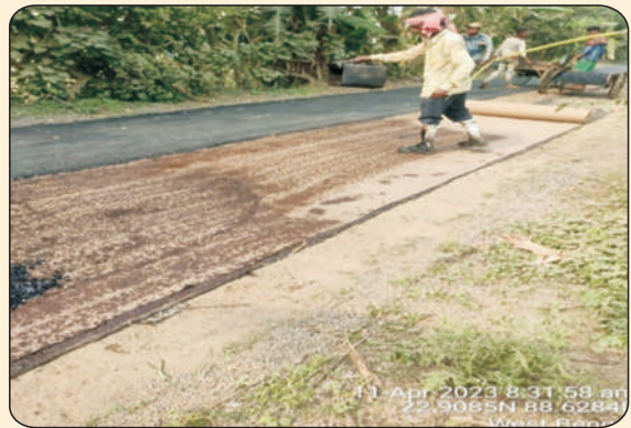
Spreading Prime & Tack Coat on JGT
