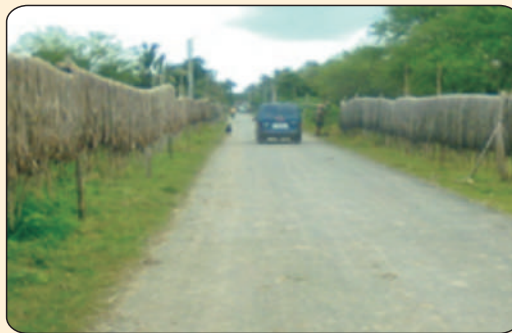
Finished Condition of road after 1 year (2015)
