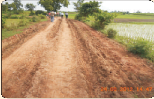
Condition of Road before construction
