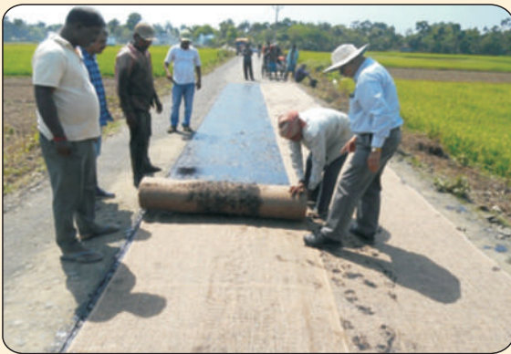
Laying of JGT
