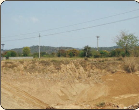
Eroded Slope of Cuttings
