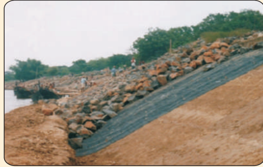
View during laying of JGT
