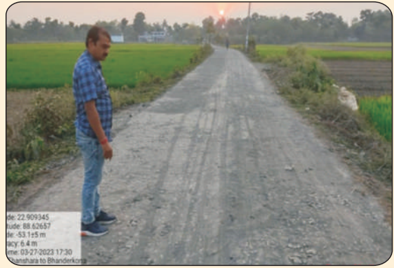
Repaired surface of damaged road
