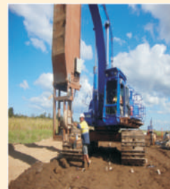
PVJD installation in progress at Ballina, Australia
