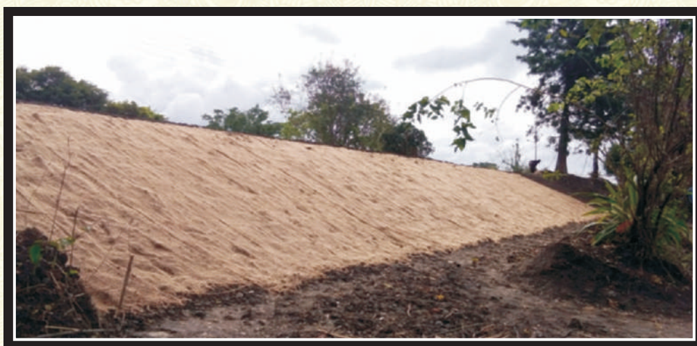
Slope Protection with JGT
