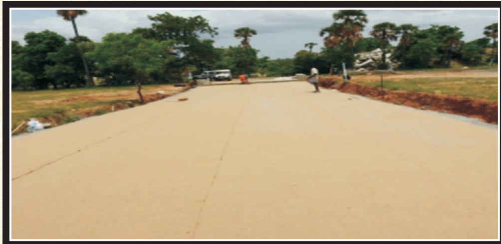
Road Construction with JGT
