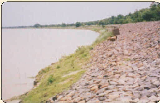
View of condition river bank after three years of JGT application
