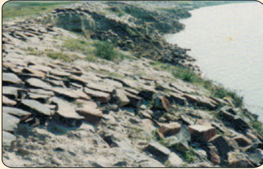
View of Eroded River Bank
