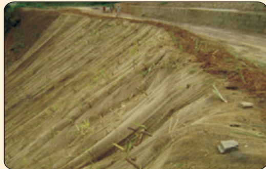
Installation of JGT
