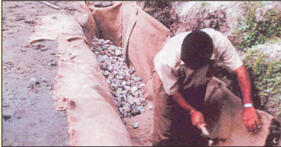
Non woven jute geotextile as trench drain
