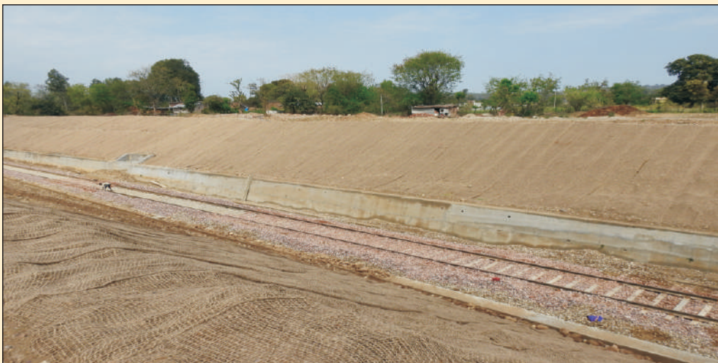
JGT Laid over the prepared slope
