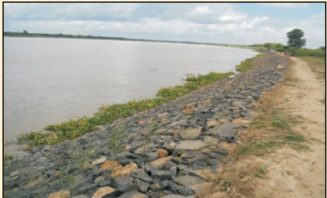
Jute geotextile treated stabilized river bank
