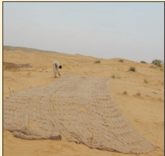
Laying of JGT
