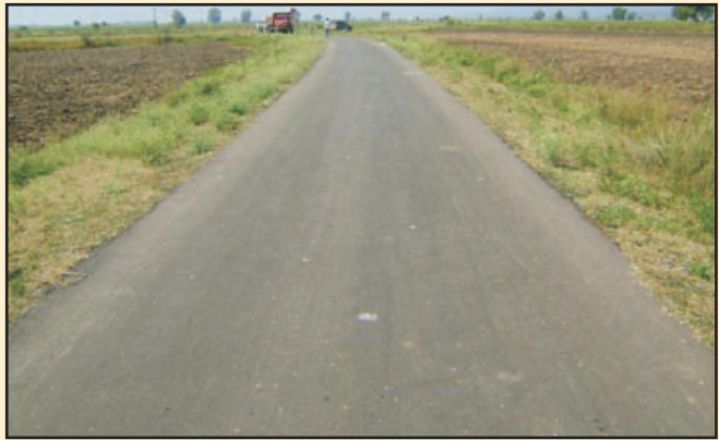
Road constructed with jute geotextile
