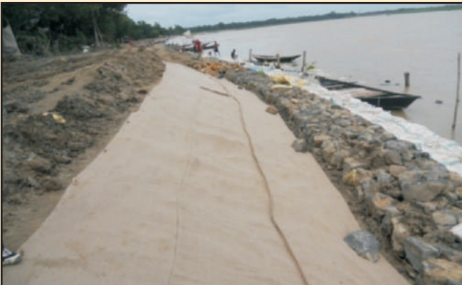
Laying of jute geotextile on eroded river bank
