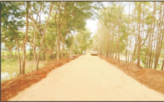
Laying of jute geotextile on road sub-grade
