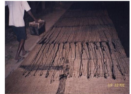
Applying tack coat on JGT
