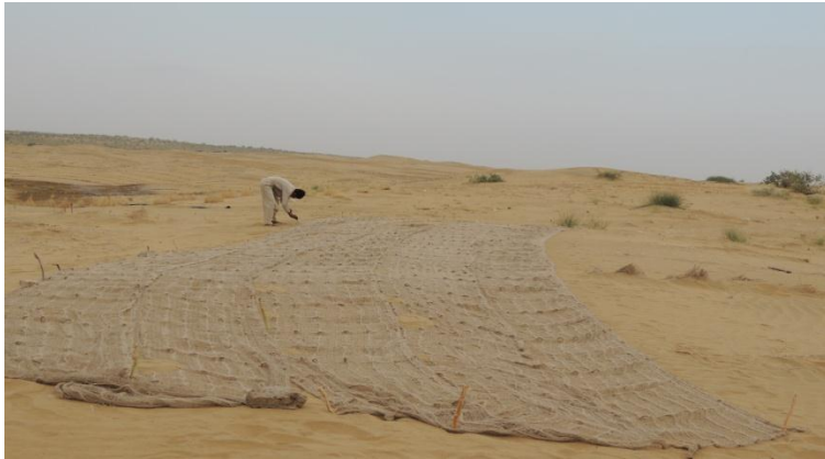
Laying of JAT
