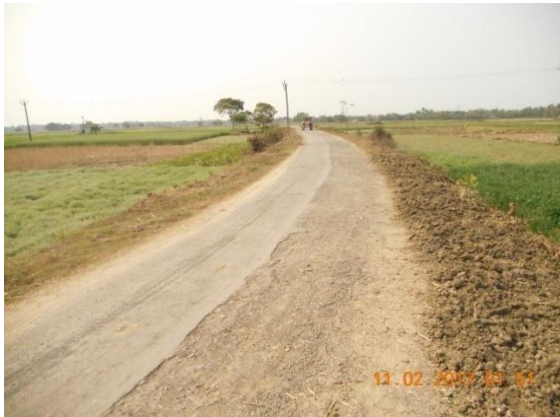
Condition of road before laying JGT
