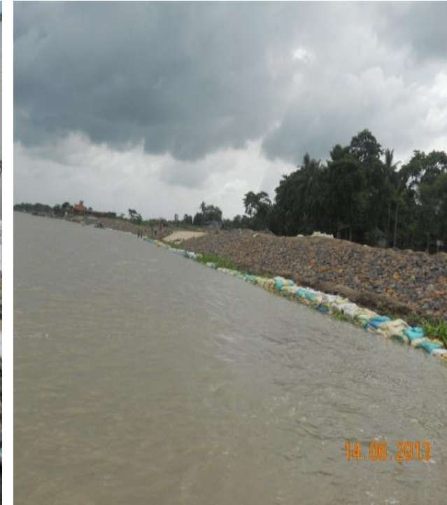
Stabilized River Bank
