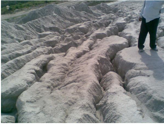
Rain cut & erosion
