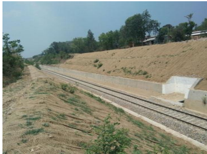
Sprouting of grass seeds through pores of JGT
