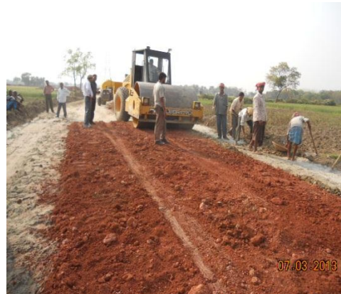
Sub-base spreading & roller compaction
