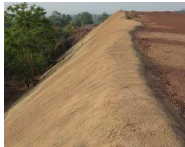
JGT laid on dressed slope
