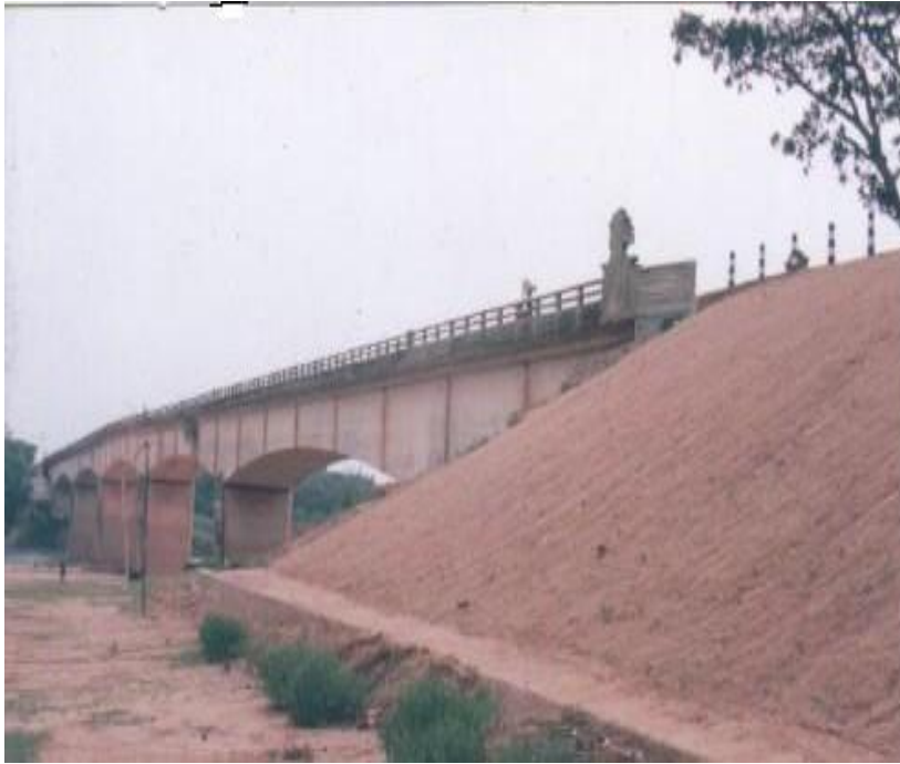
LAYING OF JGT ON THE PREPARED SLOPE
