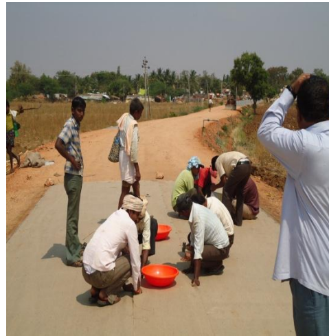
Laying of JGT on Subgrade
