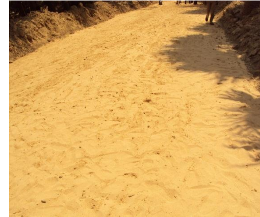
Spreading of sand over sub-grade
