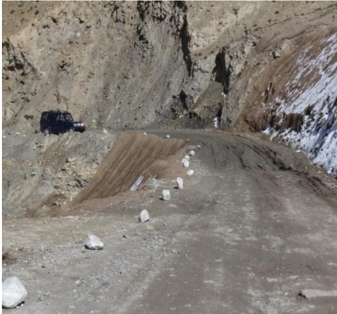
Hill slope stabilization with JGT at Ladakh - A BRO work
