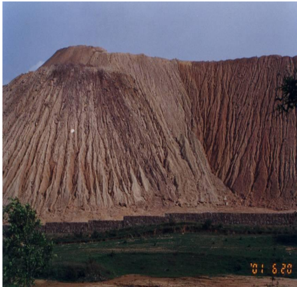
DESTABILIZED SPOIL HEAP, SINGRAULI, UP
