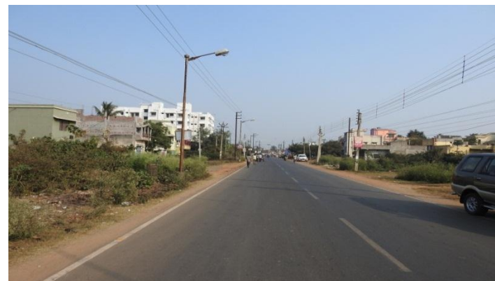
Condition of road after elapse of 3 monsoon
