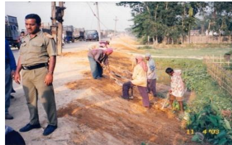
Dressing of slope for laying JGT
