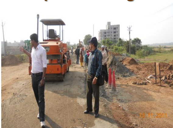
Compaction of GSB laid over JGT
