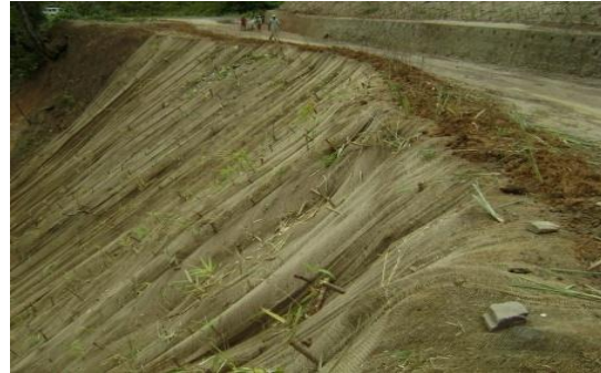
Laying of JGT
