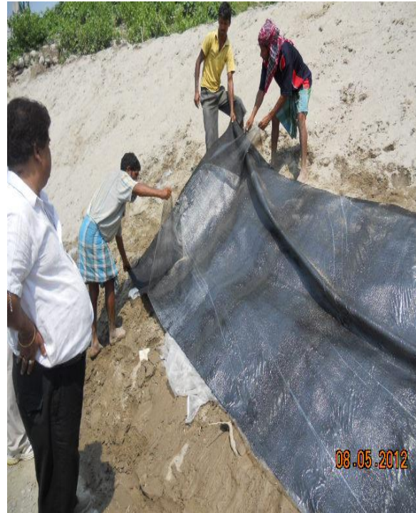
Laying of JGT on prepared bank
