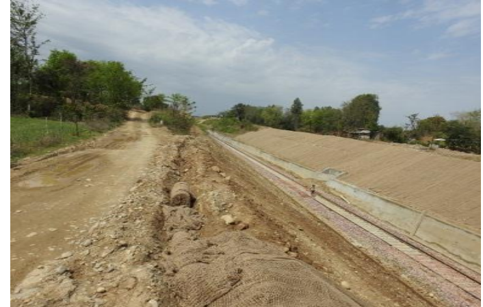
Dressing & Installation of JGT
