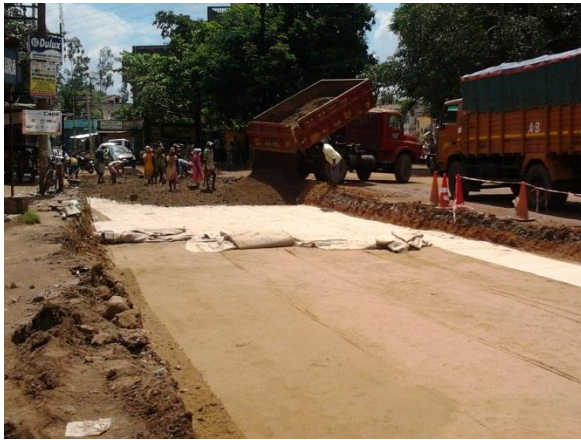
Laying of JGT on compacted sub-grade
