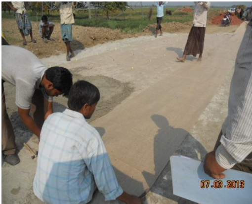
Laying of JGT with overlap
