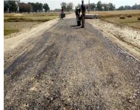
Spreading Prime & Tack Coat
