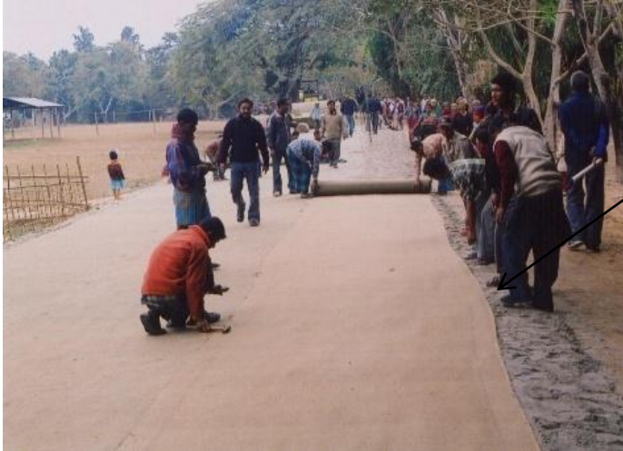
Laying of JGT & Rolling
