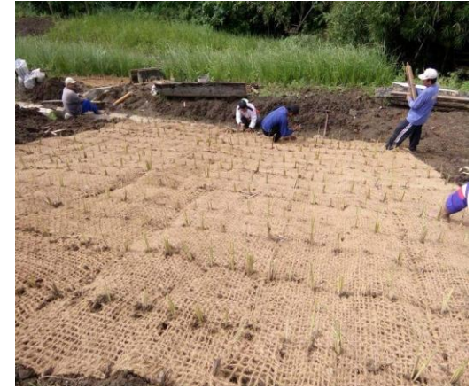
JGT laid on Slope
