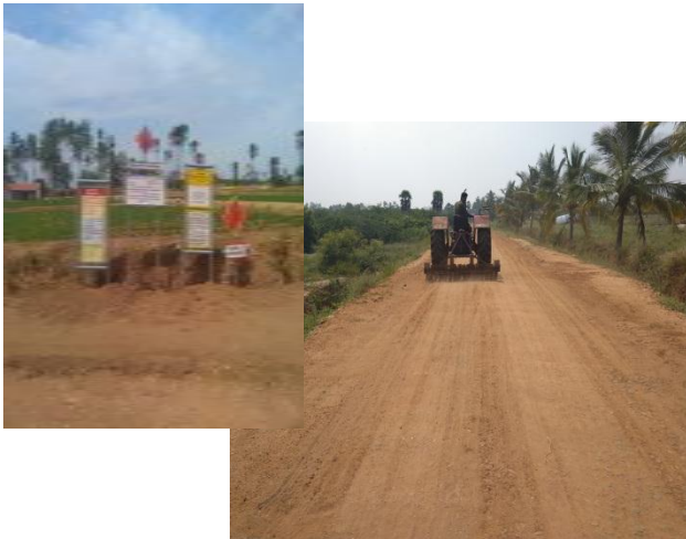
Signage & preparation of road Sub-grade
