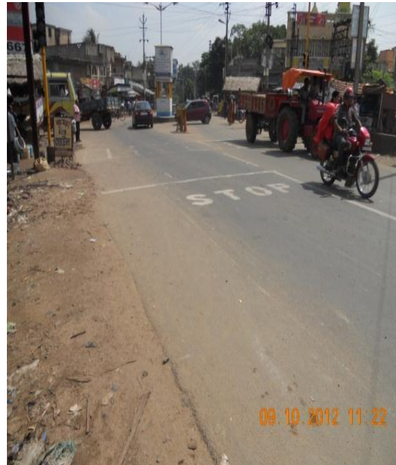
Finished Road-open to traffic
