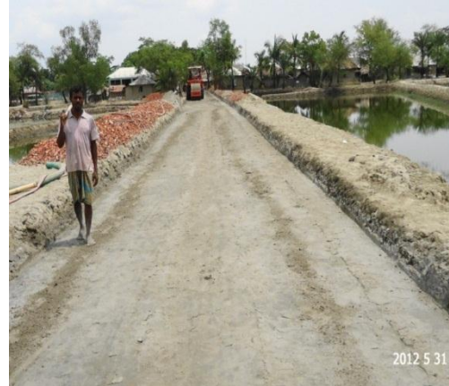
Compaction of sub- grade with roller
