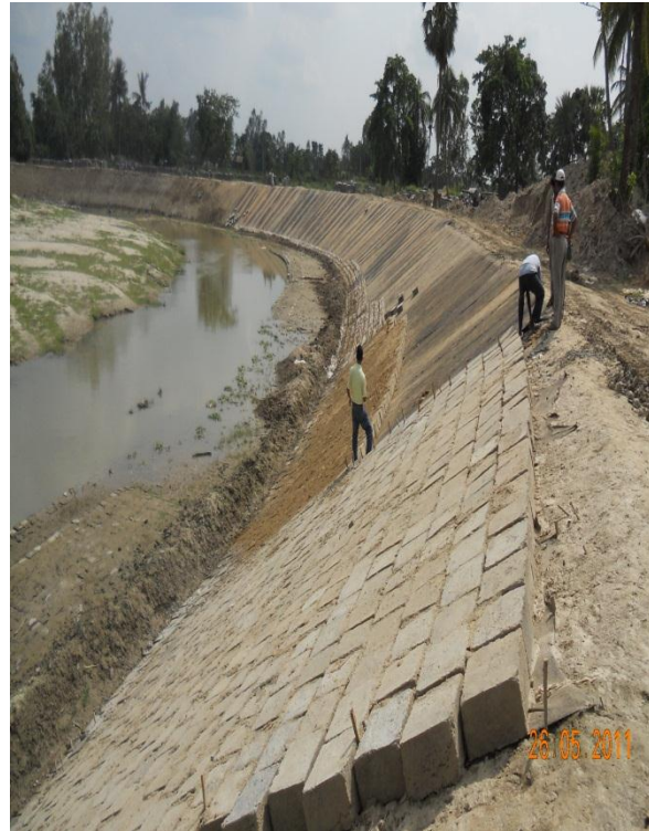
Armoring over JGT laid on bank
