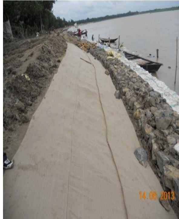
Installation of JGT
