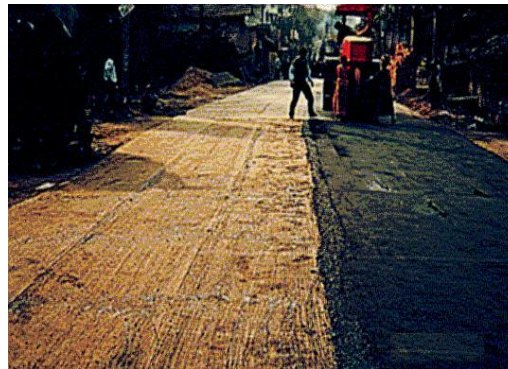
Roller Compaction of PMC
