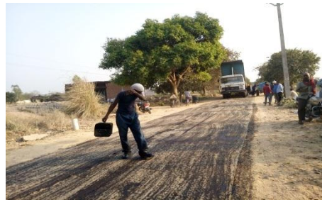
Spreading Prime & Tack Coat on JGT
