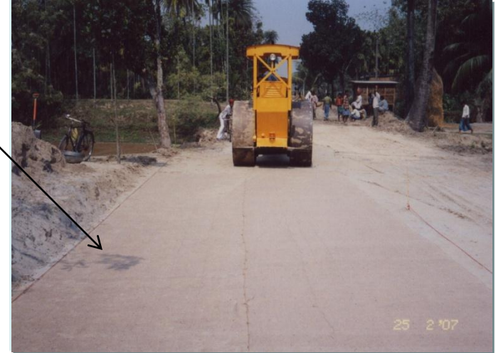
Laying of JGT & Rolling
