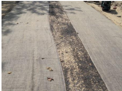
Laying of JGT
