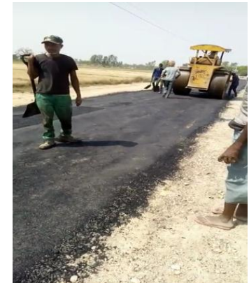
Seal Coating and Compaction
