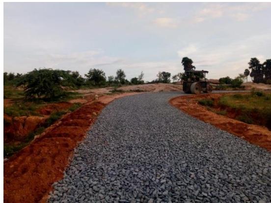
Compacted GSB laid over JGT
