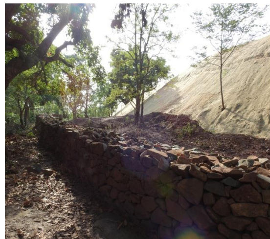
Gabion at Toe
