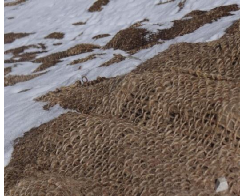
Stabilized hill slope and formation of ice on JGT
