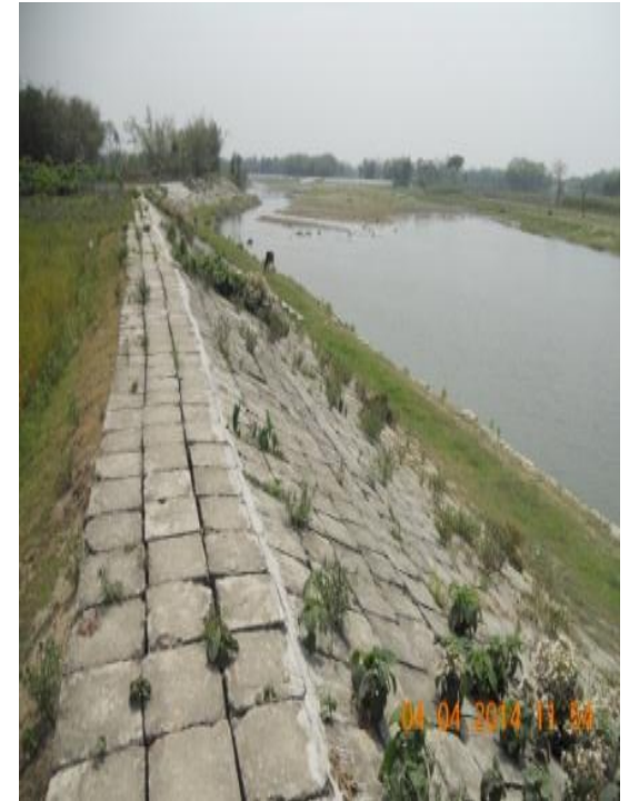
Stabilized River Bank
