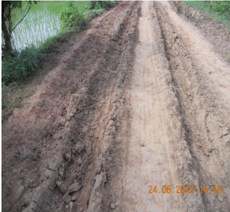
Pre-work Condition of Road
