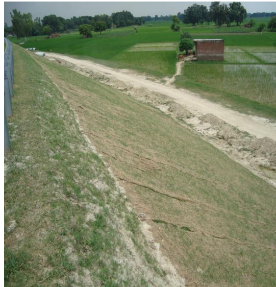
Slope protection of road through bio-engineering technique
