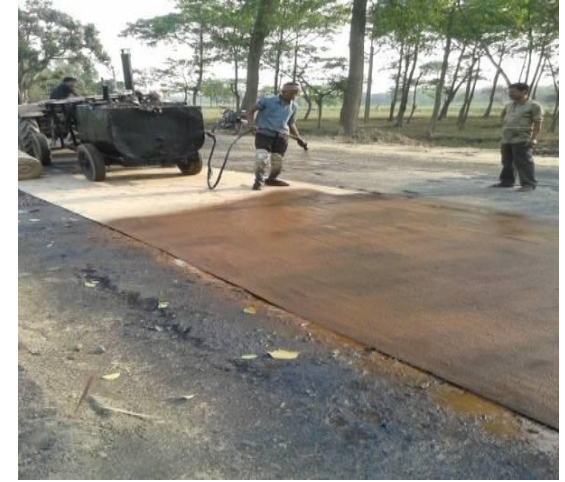
Tack coat application
