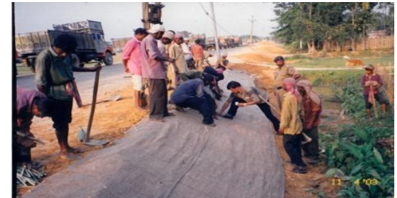
Laying of JGT
