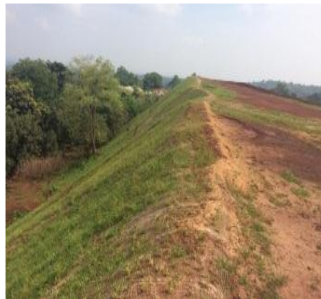
Slope Stabilized with vegetative growth
