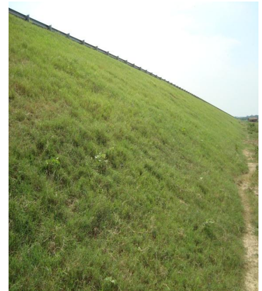
Slope protection of road through bio-engineering technique
