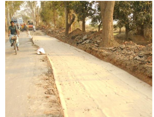
Laying of JGT on compacted sub-grade
