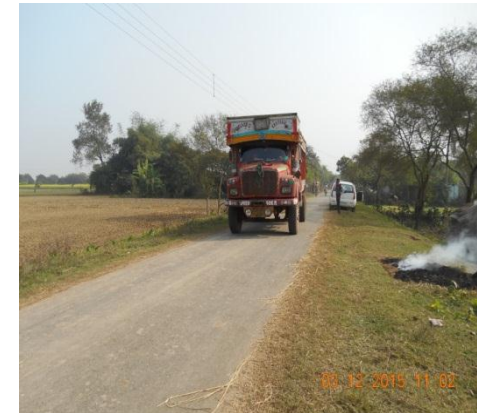
Condition of road after two years
