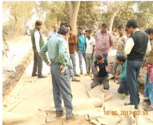
Laying of JGT on compacted sub-grade
