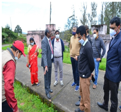
Slope protection with JGT
