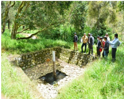
Use of nonwoven JGT in ground water recharging
