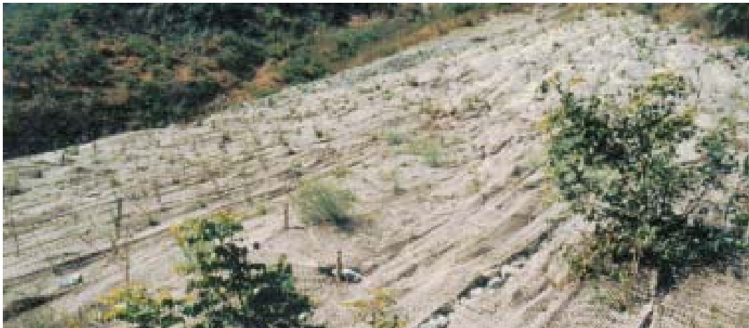
JGT laid over the prepared slope, Shahasradhara
