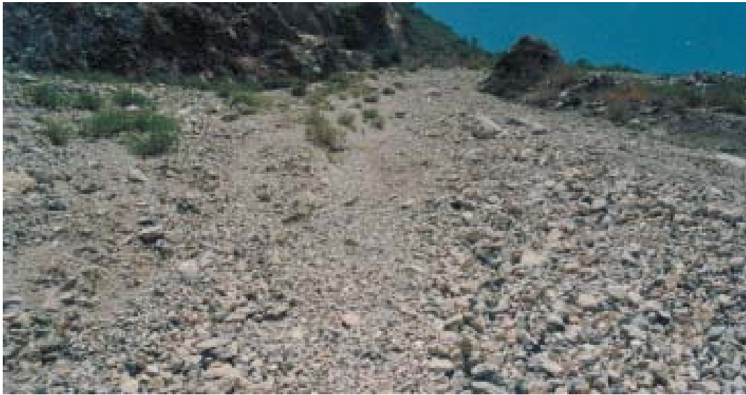
Destabilised hill slope, Sahashradhara
