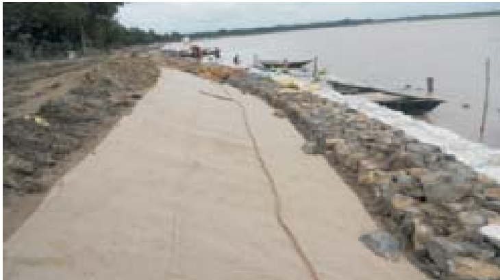
◀ LAYING OF JUTE GEOTEXTILE ON ERODED RIVER BANK
