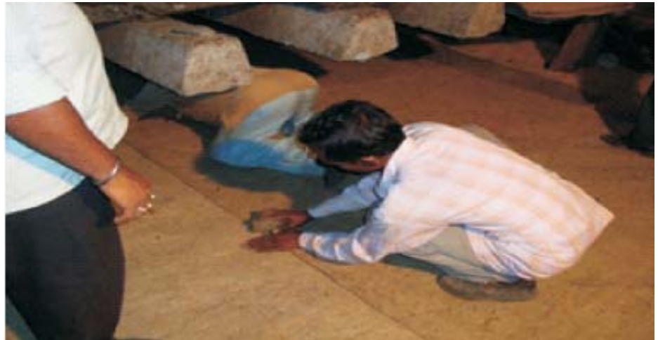
NONWOVEN JUTE GEOTEXTILE LAID ON THE ▶ FORMATION OF RAILWAY TRACK
