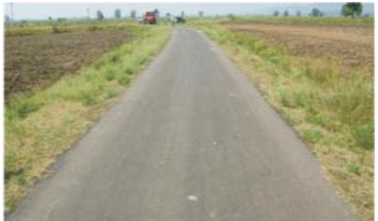
ROAD CONSTRUCTED WITH JUTE GEOTEXTILE ▶
