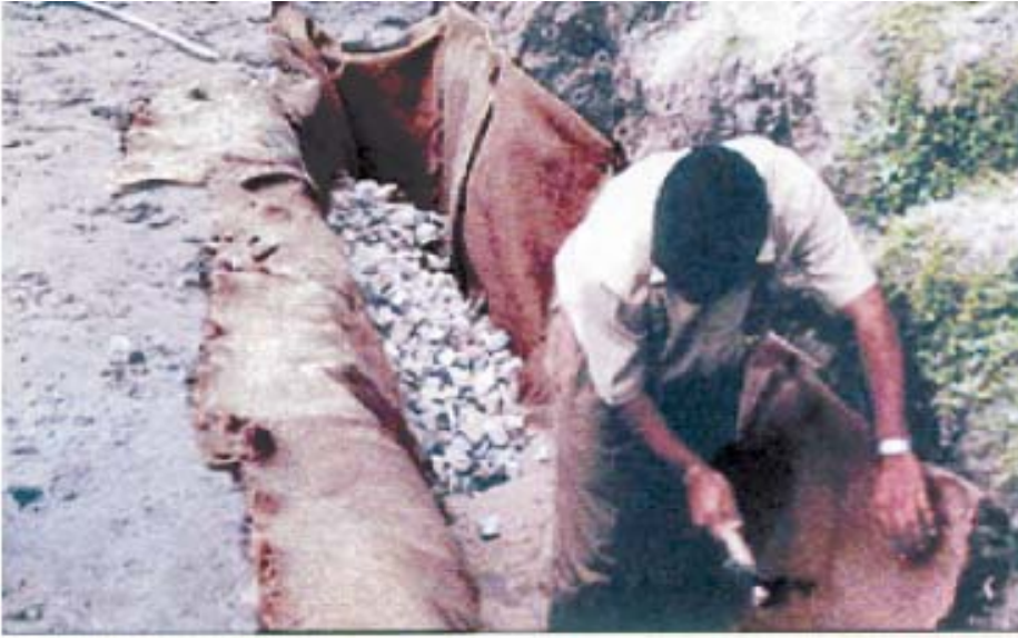
NON WOVEN JUTE ◀ GEOTEXTILE AS TRENCH DRAIN
