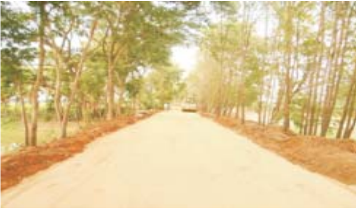
◀ LAYING OF JUTE GEOTEXTILE ON ROAD SUB-GRADE
