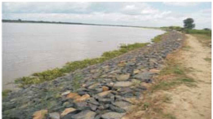
JUTE GEOTEXTILE TREATED STABILIZED RIVER BANK ▶
