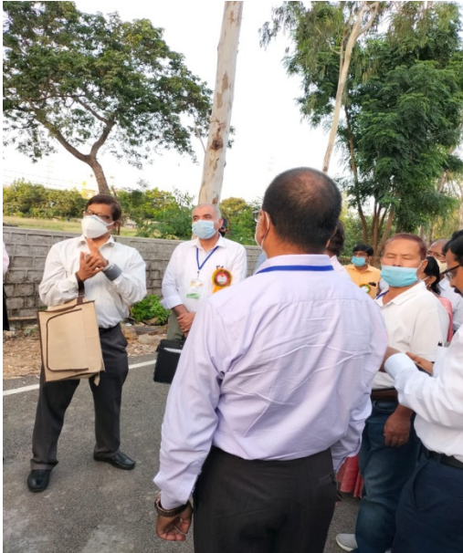
Explaining the efficacy of JGT by NJB to the delegates in road construction works
