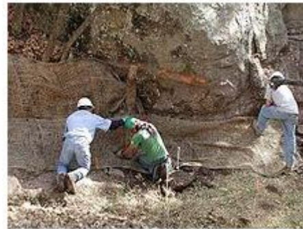
Fig : 02 Use of Jute Matting
