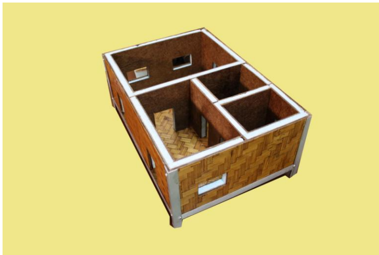
Model Emergency Shelter from Sandwich Panel
