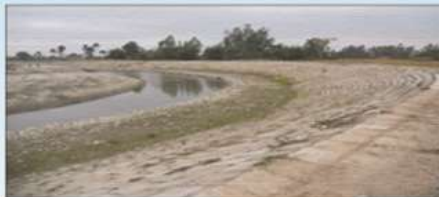
STABILIZED RIVER BANK PREPARED WITH JGT
