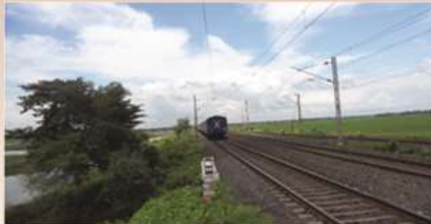
FINISHED TRACK (AFTER 4 YEARS)
