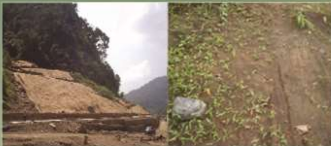
OPEN WEAVE JGT ON THE AFFECTED SLOPE
