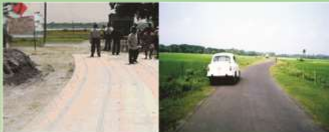
JGT LAID ON THE PREPATED SUB-GRADE OF ROAD
