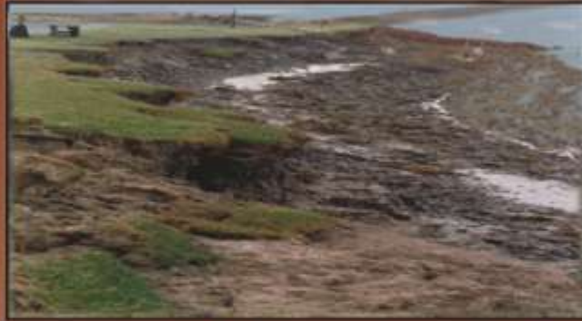
ERODED BANK OF NAYACHAR HOOGLY, 1998
