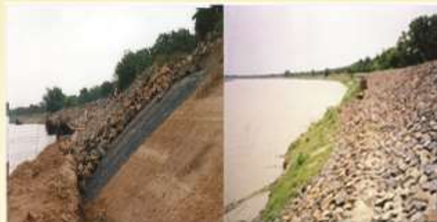
LAYING OF JGT AND RIP RAP ON SLOPE
