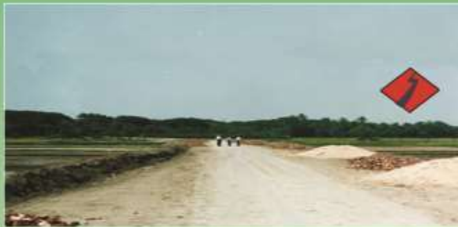
PREPARED SUB-GRADE BEFORE LAYING JGT
