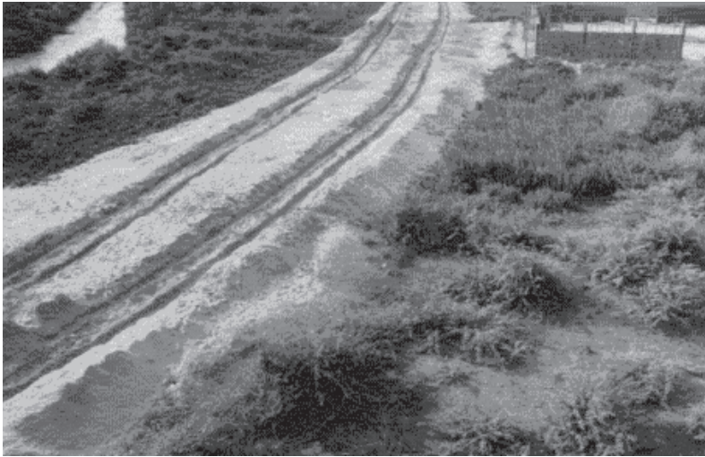
Fig. 11 Embankment construction nearing completion
