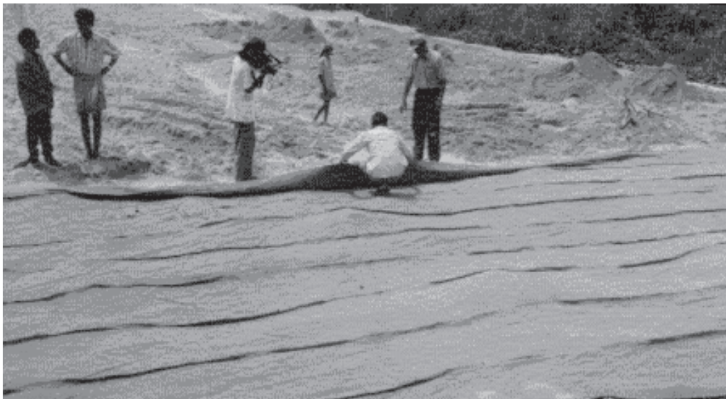
Fig. 8 Woven jute geotextiles were laid over the soft ground
