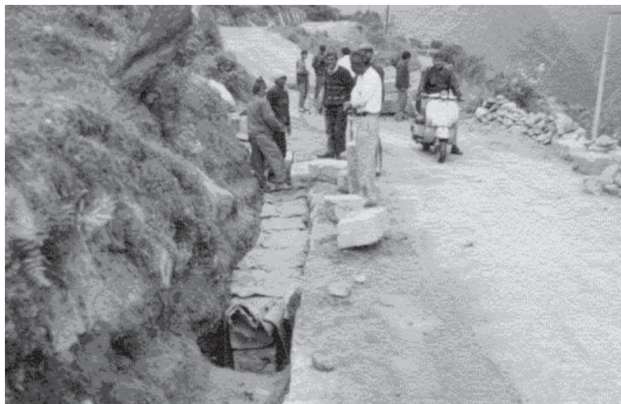
Fig. 3 Rubbles encapsulated in jute geotextile.
