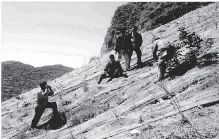
Laying of JGT at Kaliasaur land slide, HP Sirmaur
